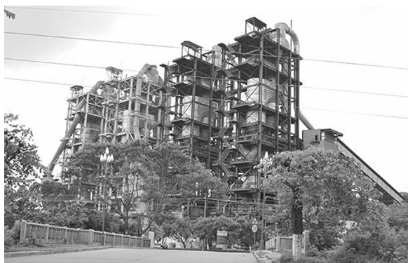
Figure 1. The evaporators in AEP.
